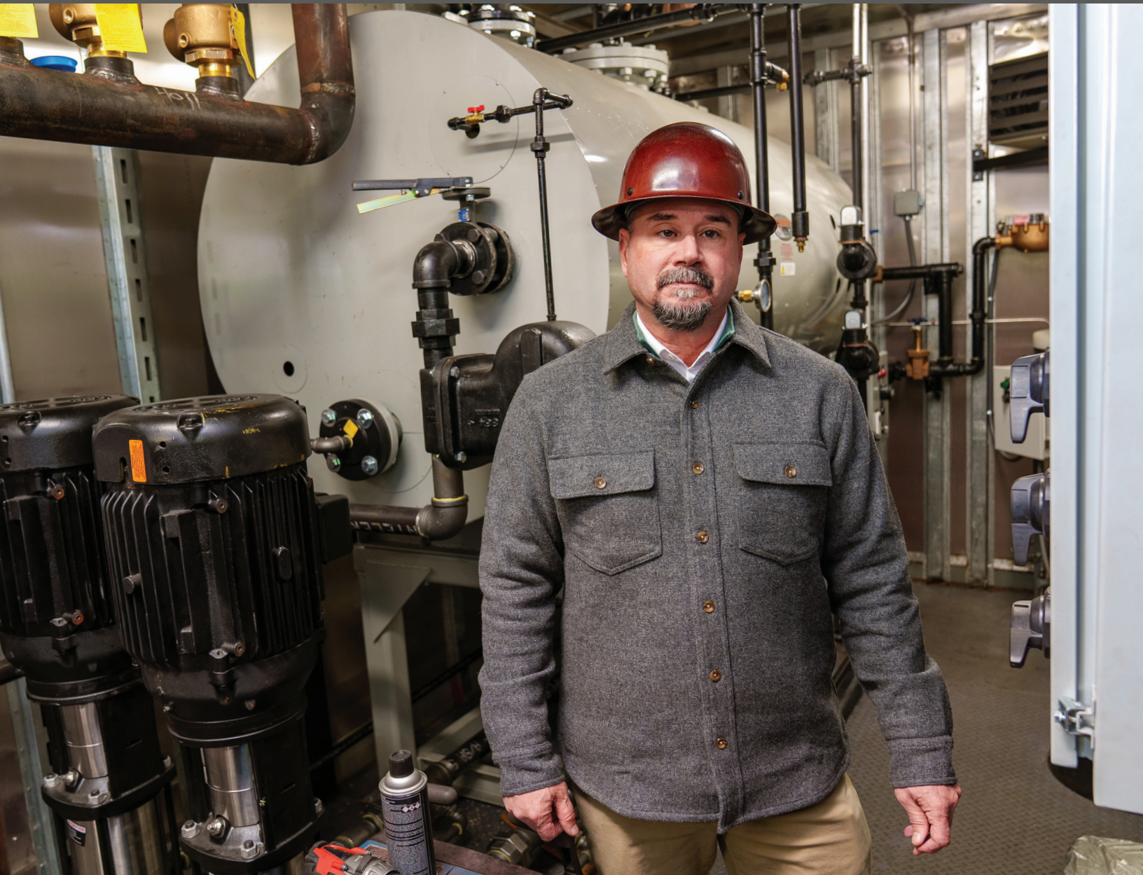
Jim Cipollone leads Burnham's new rental boiler affiliate, Thermal InMotion, which provides a variety of mobile boiler rooms for short and long term rental
