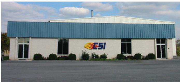
CSI offices, service shop and fabrication plant in York, PA
